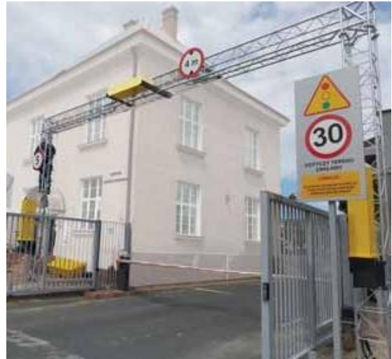
PI-MSKA system with an upper detector and two detectors positioned opposite each other
